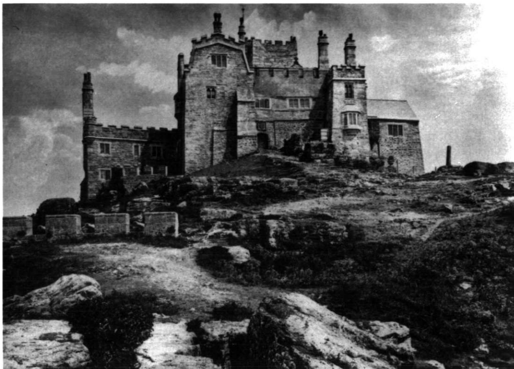
Fig 1 The early 20th century Gibson photograph of the west end of St Michael's Mount summit complex. Imagine away the 19th century extension to the north (left), the mansard gable on the large tower to the north of the door, all the chimneys, and Piers St Aubyn's pseudo-medieval windows, and the sturdy later medieval castle re-emerges. Poking up behind, itself battlemented, is the priory church's tower, with the fragment of medieval lighthouse on its south-west (right) corner. The remains of a medieval curtain wall were recorded curving from behind the 18th century battery in the foreground to the cross-shaft (right); this protected the long flight of steps running up to the castle. (Courtesy of the Royal Institution of Cornwall).
