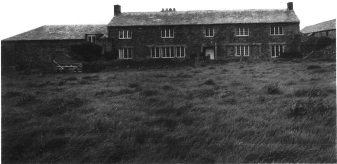
Fig 8 Stowe Barton farmhouse from the south. (RCHME Crown Copyright)
