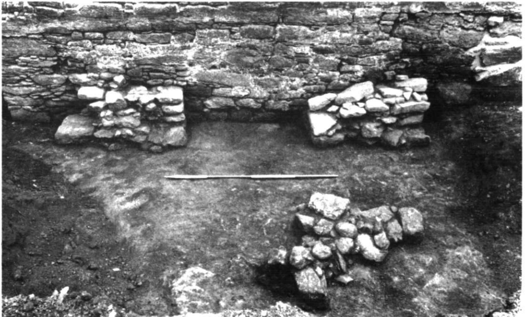
Fig 15 The three surviving foundation fragments of the former north tower, exposed during drainage and landscaping works. (Photo: Warwick Rodwell)
