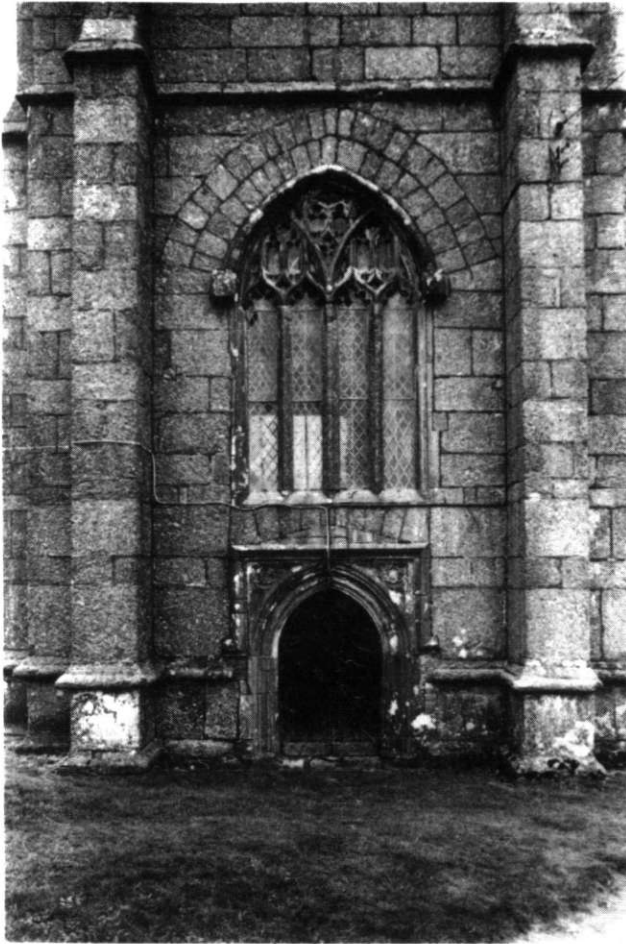
Fig 18 Ground stage of the west tower, showing the modest doorway and large window with uncarved label-stops. (Photo: Warwick Rodwell)
