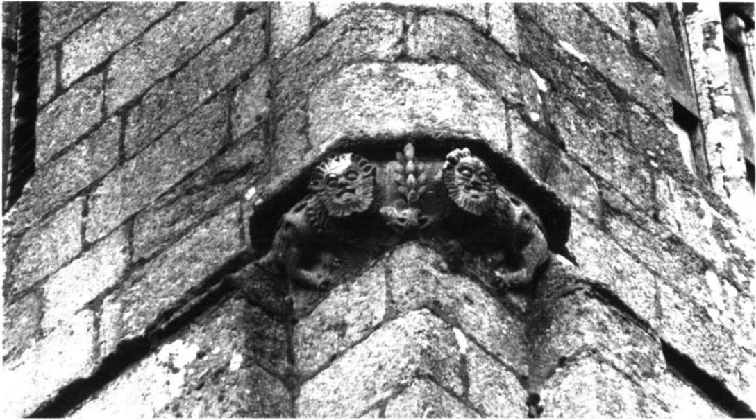
Fig 20 Sculptured corbel supporting the south-west corner turret of the tower. (Photo: Warwick Rodwell)
