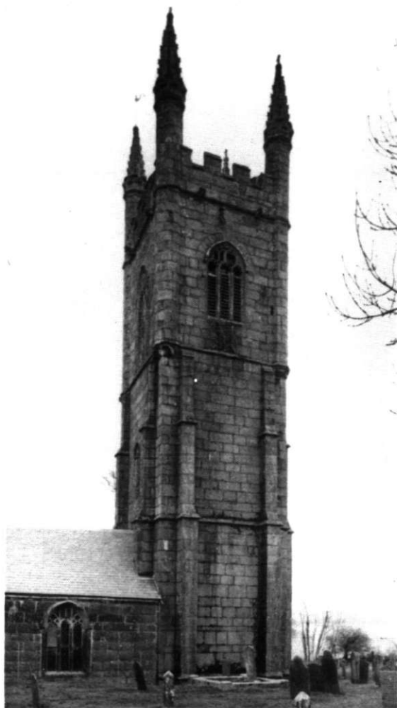
Fig 17 West tower and nave abutment, viewed from the north. (Photo: Warwick Rodwell)
