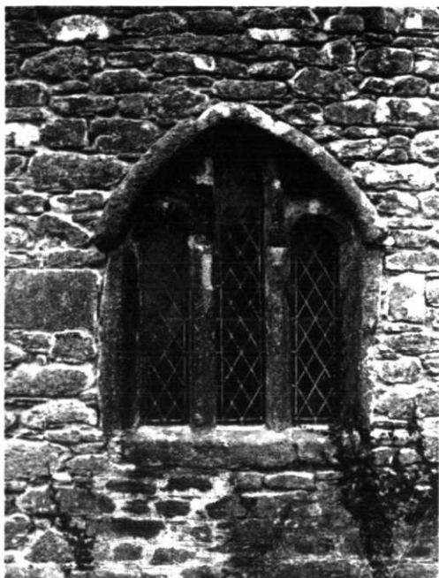
Fig 11 Simple triple-lancet window in the east face of the north transept, the earliest extant architectural feature in the church. (Photo: Warwick Rodwell)
