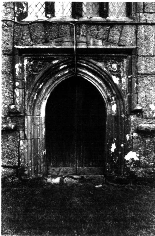
Fig 19 Detail of the west doorway with its heavy label-moulding, squat proportions, and uneasy relationship to the tower plinth. (Photo: Warwick Rodwell)
